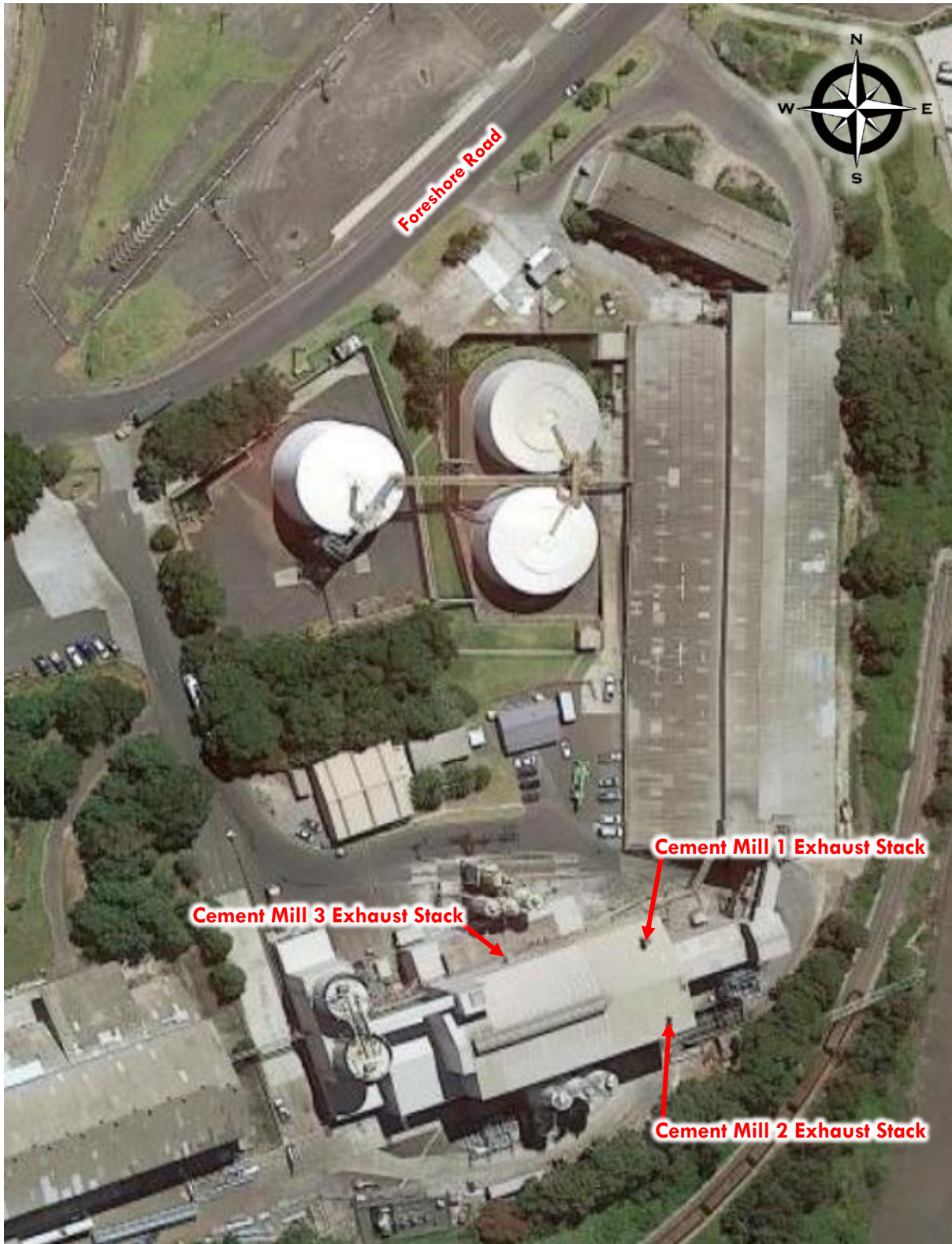
Figure 1: Cement Mill 1, 2 & 3 Exhaust Stack locations at Gate 7 Foreshore Rd, Port Kembla, NSW
