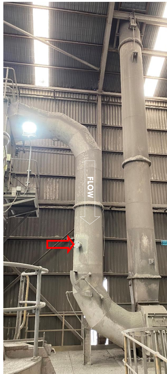
Figure 2: Cement Mill 1 Exhaust Stack sampling plane location
