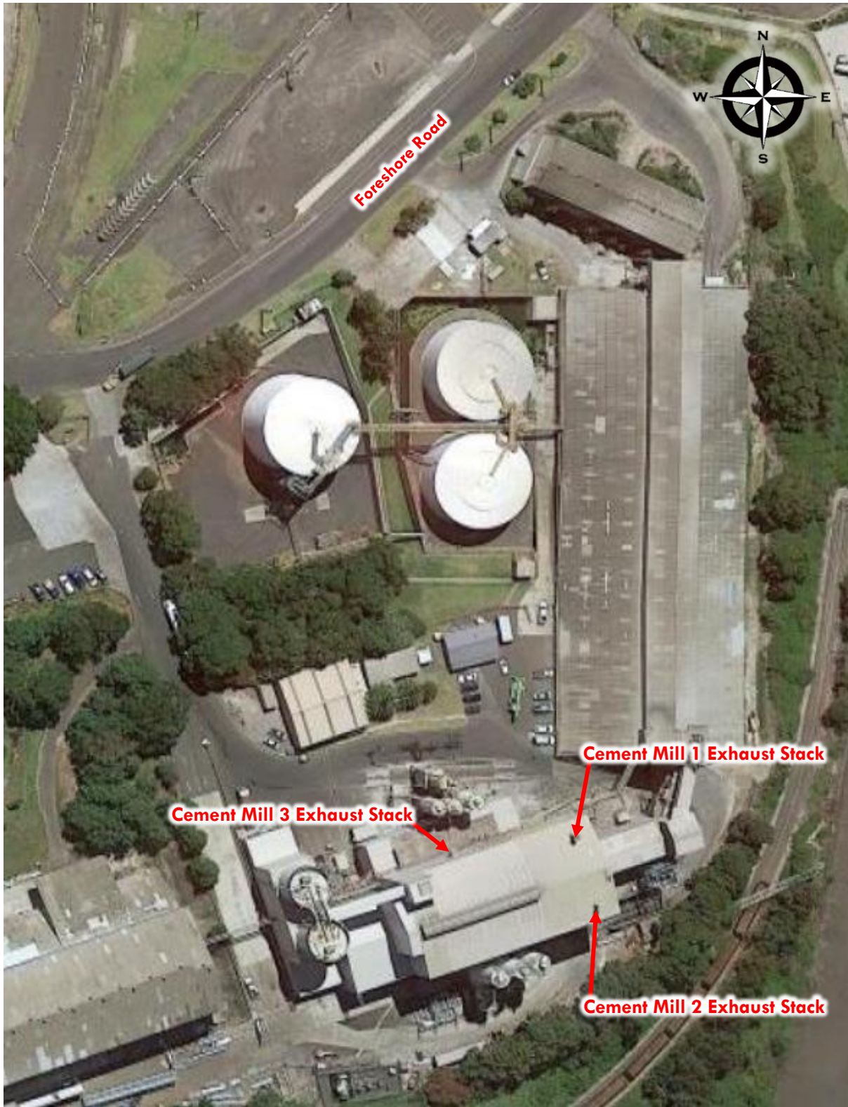
Figure 1: Cement Mill 1, 2 & 3 Exhaust Stack locations at Gate 7 Foreshore Rd, Port Kembla, NSW
