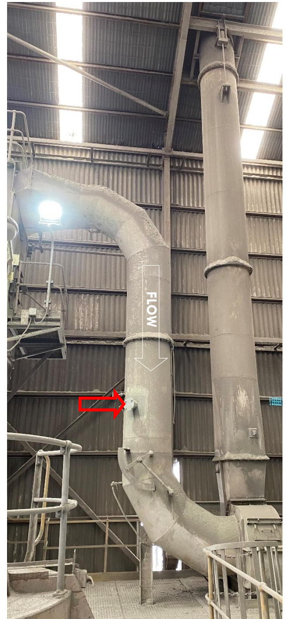
Figure 2: Cement Mill 1 Exhaust Stack sampling plane location.
